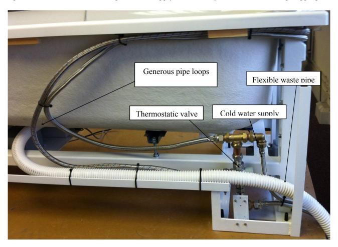
If pipe-work is not supplied, or the installation is modified, it is important to ensure that the above layout is maintained, with generous pipe loops to ensure that the pipe-work is not under any strain during raising and lowering of the bath. These should be positioned in the space along the side of the bath, between the bath wall and the panels.
